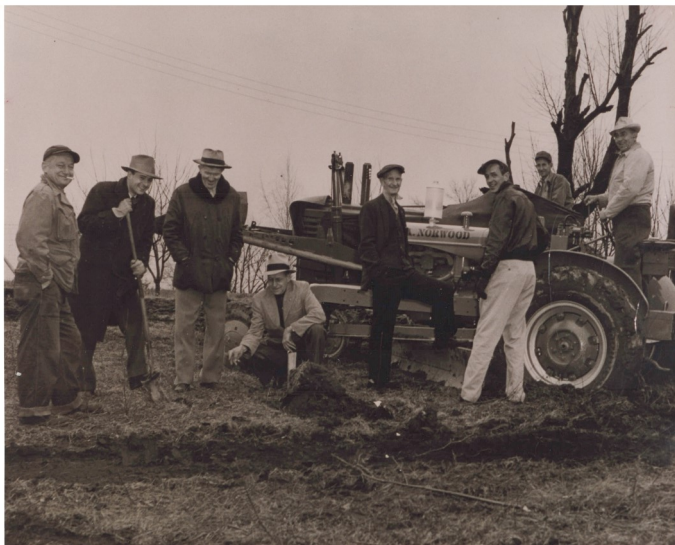
Ground Breaking January 28th, 1950, Cost $22,000
